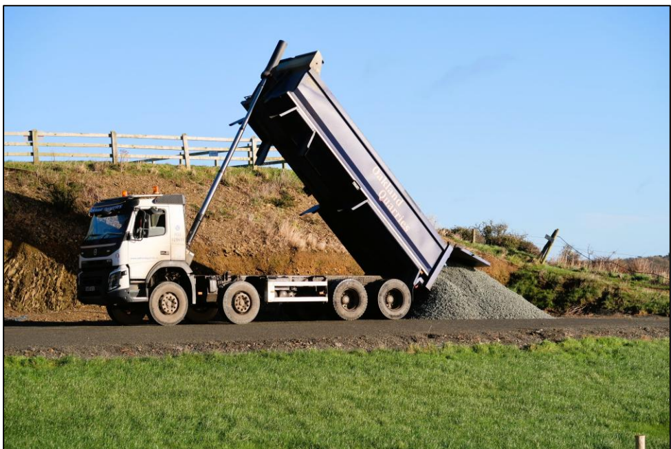
Plate 11. Crushed stone being delivered to surface the shelf.
